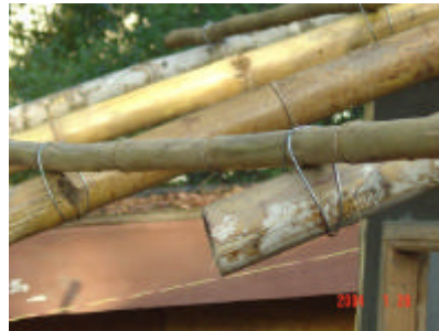
Pictures 29: Fixing purlins
