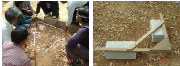
Picture 8: using 3-4-5 method to fix the corners of the building
