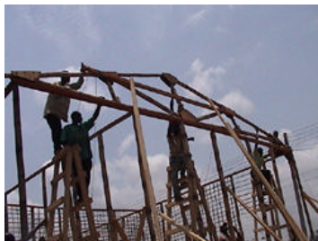
Pictures 25-26: Truss hanging and fixing
