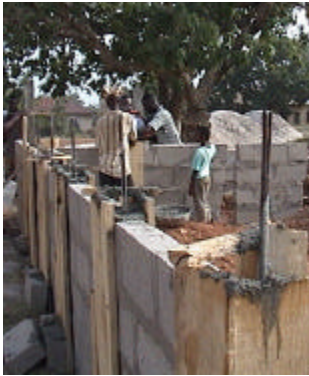
Picture 11-12: Foundation column and ground slab
