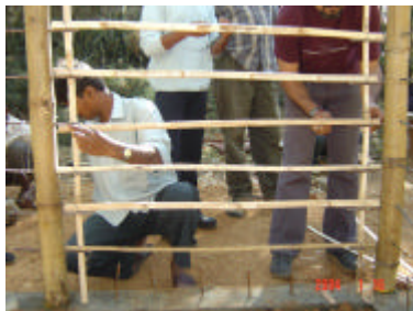
Picture 18-19: Bamboo wall grids
