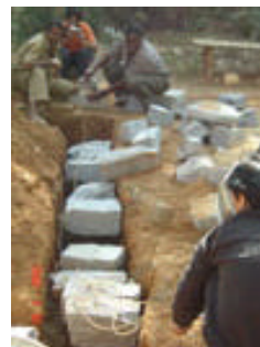
Picture 9: Levelling by transparent water pipe
