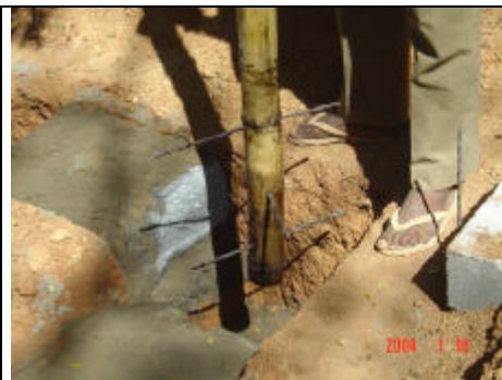
Picture 13: Foundation to embed columns
