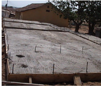
Picture 11-12: Foundation column and ground slab
