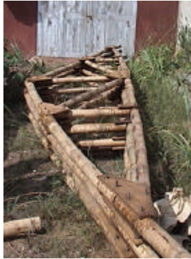
Pictures 23-24: Trusses and a joint
