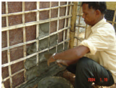
Picture 21-22: Rough and smooth plastering
