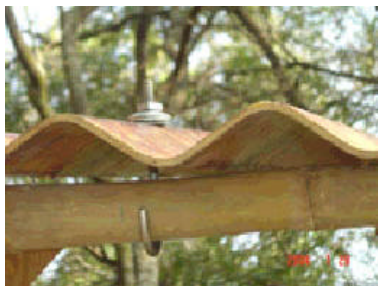
Pictures 30-31: L Fixing roof cover
