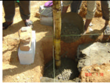
Picture 15: Embedding bamboo column
