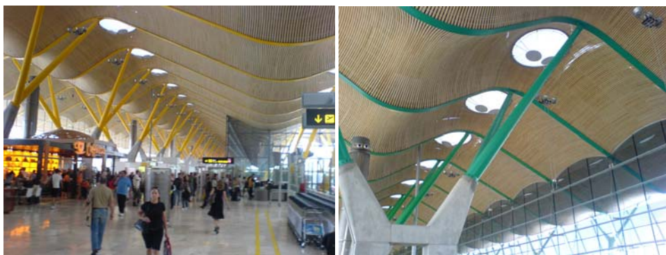
Figure 4.2: In the ceiling of the new airport terminal in Madrid by Richard Rogers, the bendability of plybamboo laths is utilized
