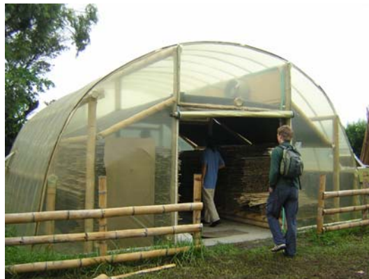
Figure 2.3: Low cost solar powered drying chamber for bamboo strips in Colombia developed by Jörg Stamm
