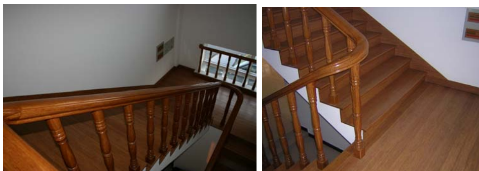
Figure 1.8: Application of SWB in a stairway
