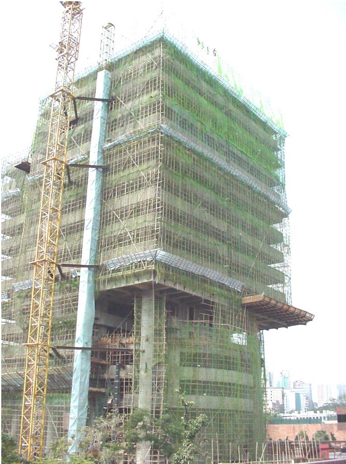
Figure 1.1 Typical bamboo scaffold – Double Layered Bamboo Scaffold (DLBS)
