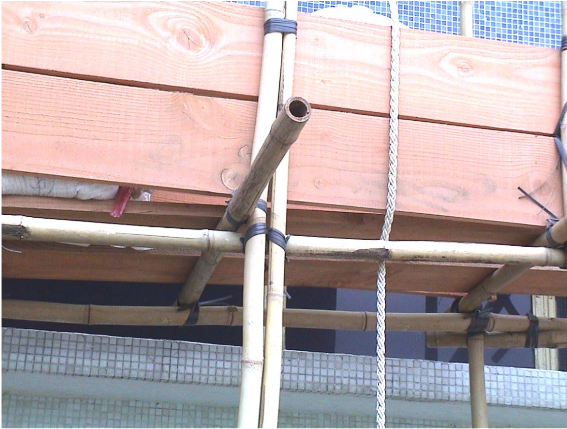
Figure 1.4 A close-up on the ledger-post connection
