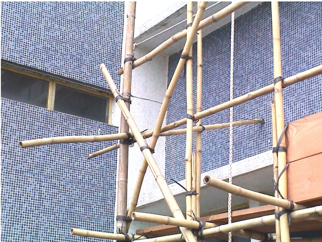
Figure 1.5 Detail of a putlog attaching the post of the outer layer in a DLBS
