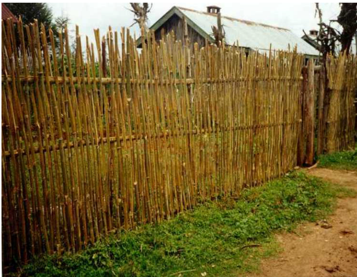
Plate 7: A newly constructed bamboo fence at Timboroa
