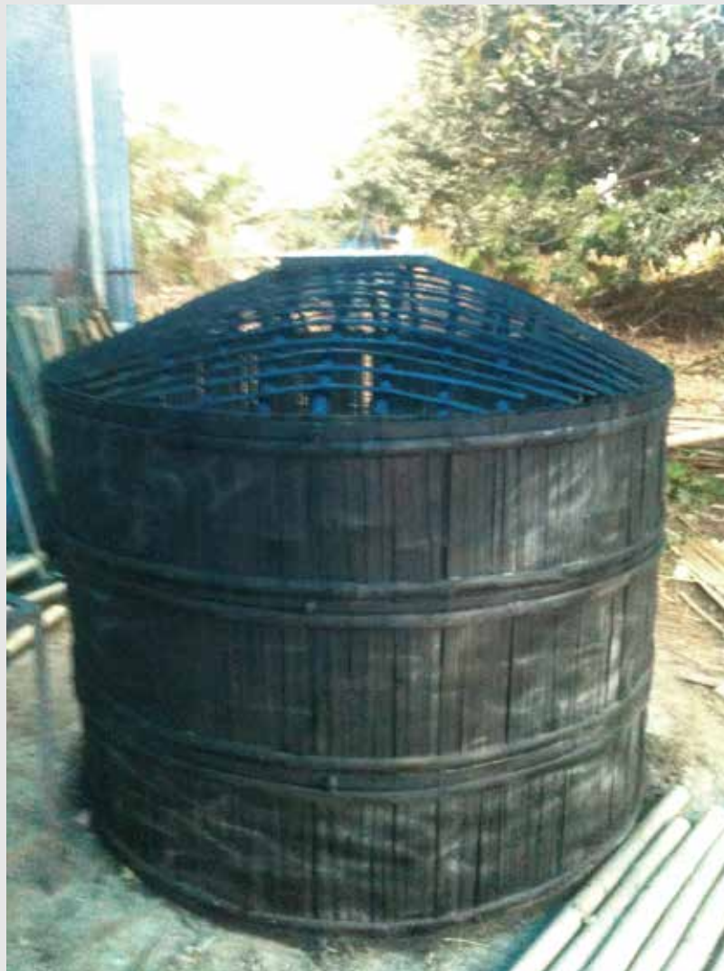
Figure 27: Application of bitumen coating
