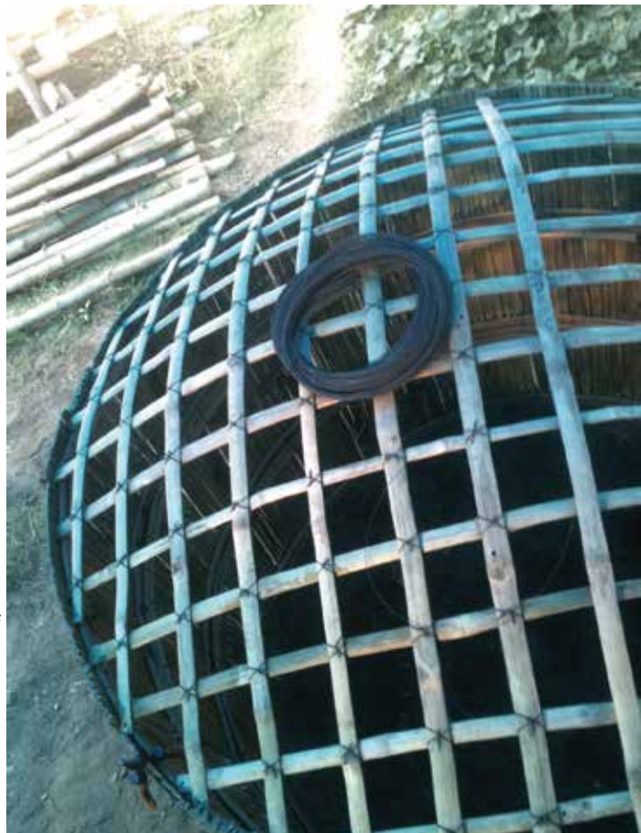
Figure 24: Attaching a grid network for dome roof
