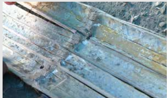
Figure 11: Interior nodes of the culm removed
