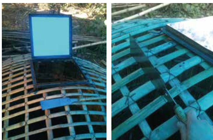
Figure 26: Cutting an opening and attaching the lid
