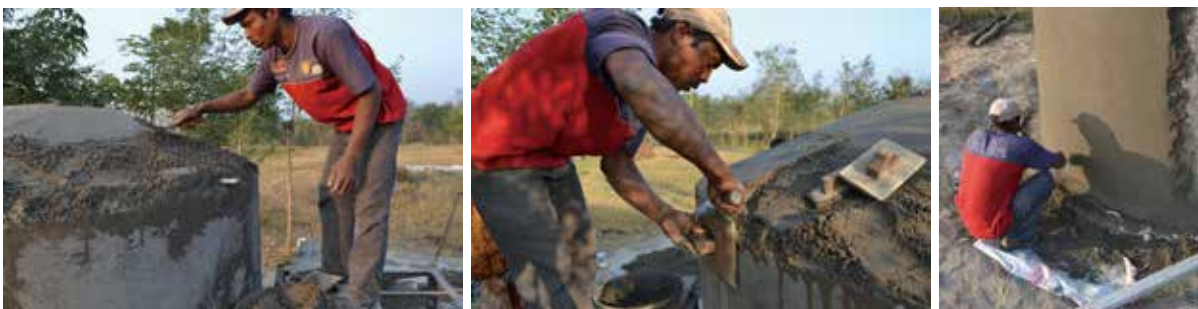
Figure 44: Roof plaster finishing and overflow pipe
