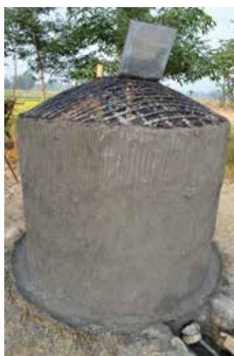
Figure 37: finished scratch coat
