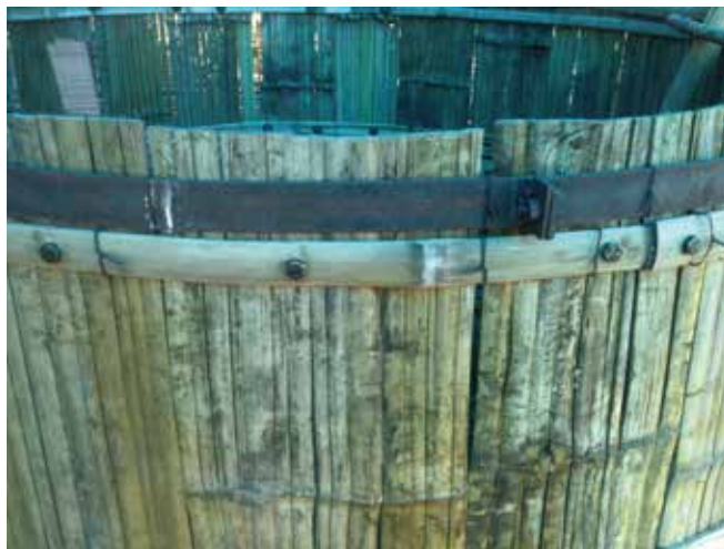
Figure 20: Bolting the bamboo strips
