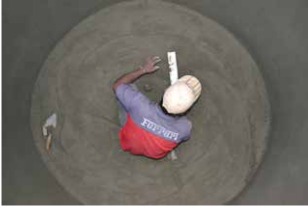
Figure 41: Floor plastering
