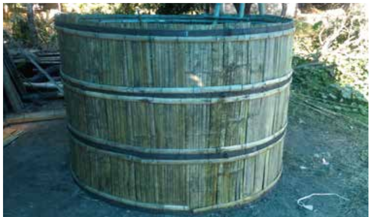
Figure 19: Attaching bamboo strips
