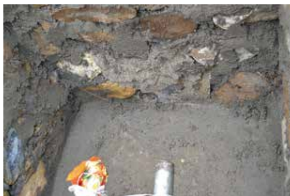
Figure 33: Drain and future pipe accommodation
