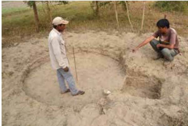
Figure 28: Site and foundation preparation
