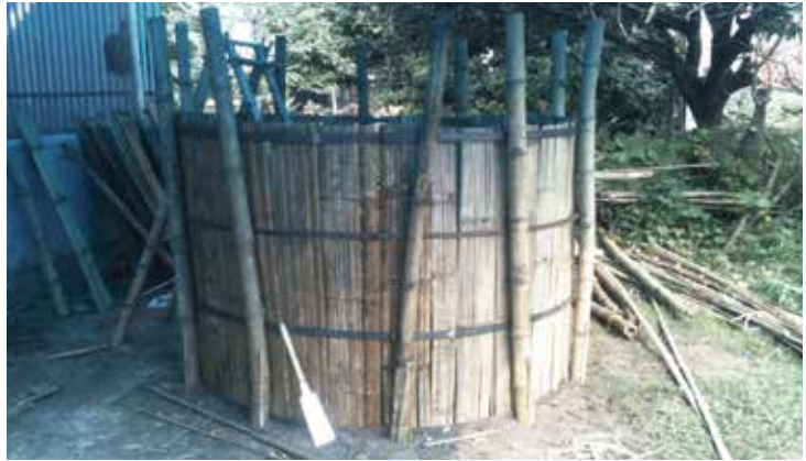
Figure 17: Finished wall with all bamboo boards attached
