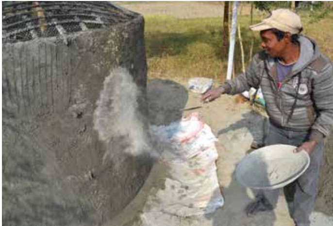
Figure 38: Final exterior coat
