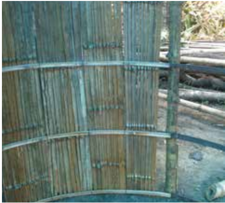
Figure 16: Fitting bamboo board with half the wall finished
