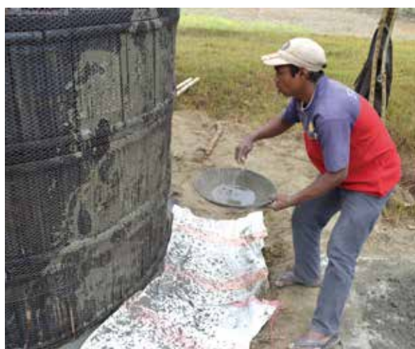
Figure 36: Application of the plaster scratch coat
