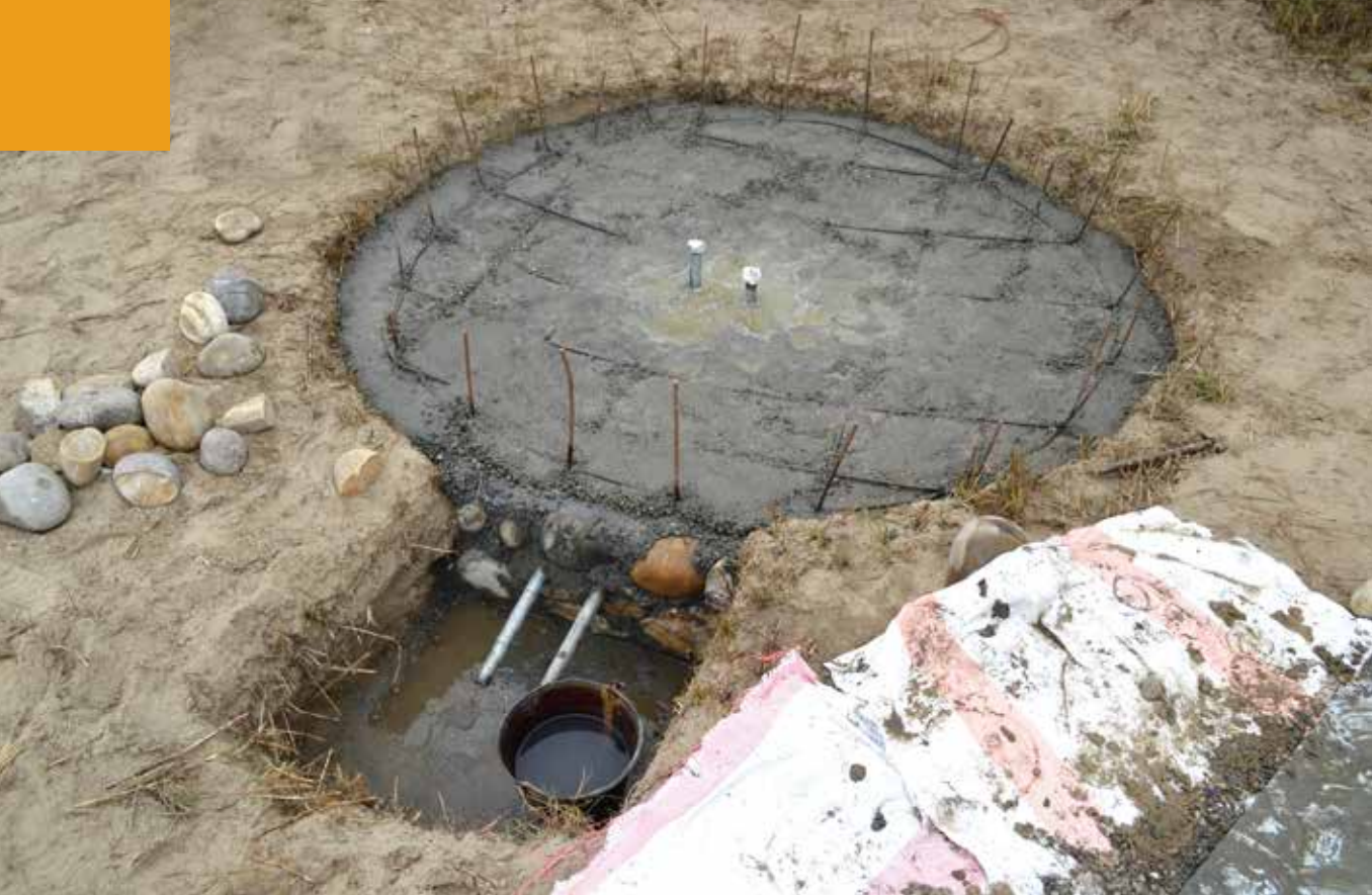
Figure 31: Pouring a concrete foundation
