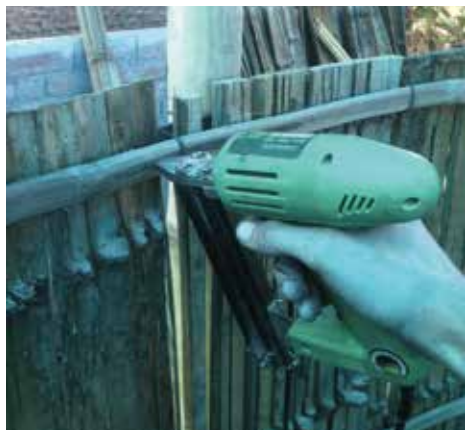
Figure 18: Stapling bamboo strips
