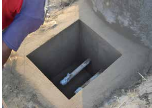
Figure 42: Access port final plastering
