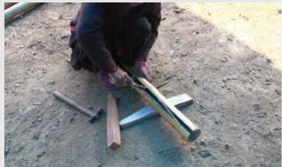
Figure 9: Splitting the bamboo open on one side
