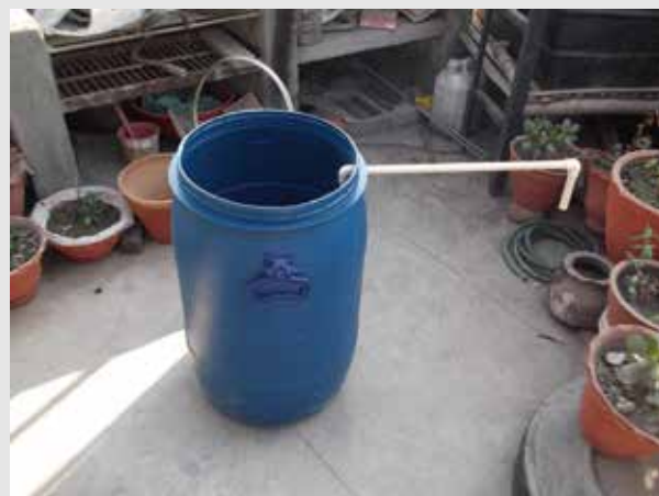
Figure 53: PVC pipe third elbow directs water outside of the tank for clean water storage
