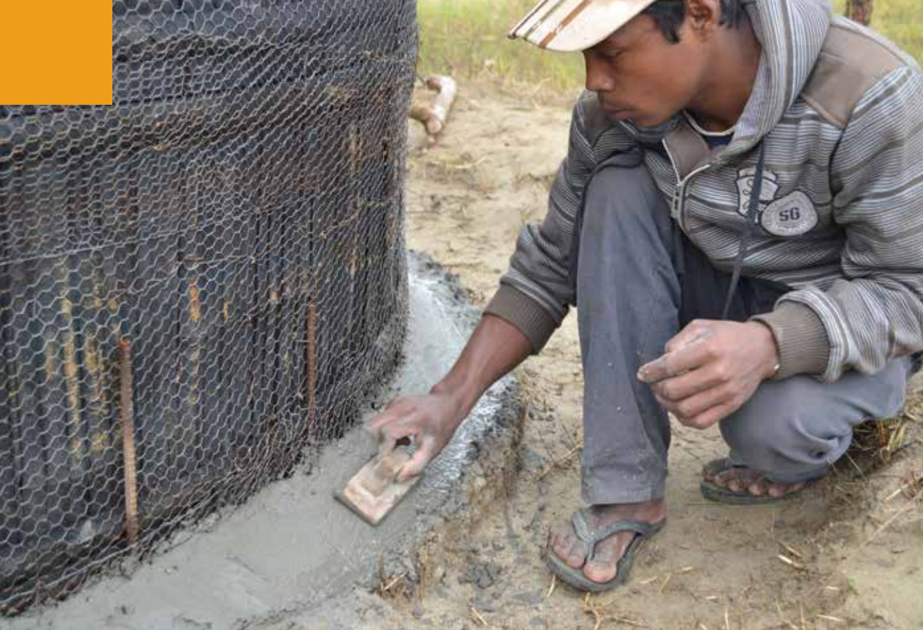
Figure 35: Concrete reinforcement at the tank base
