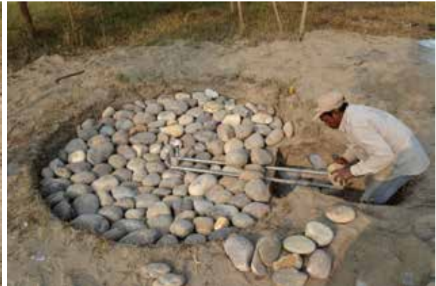
Figure 29: Fitting pipe and laying river rocks
