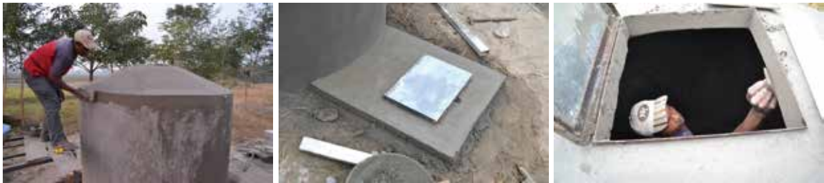
Figure 45: Completing the roof plaster
