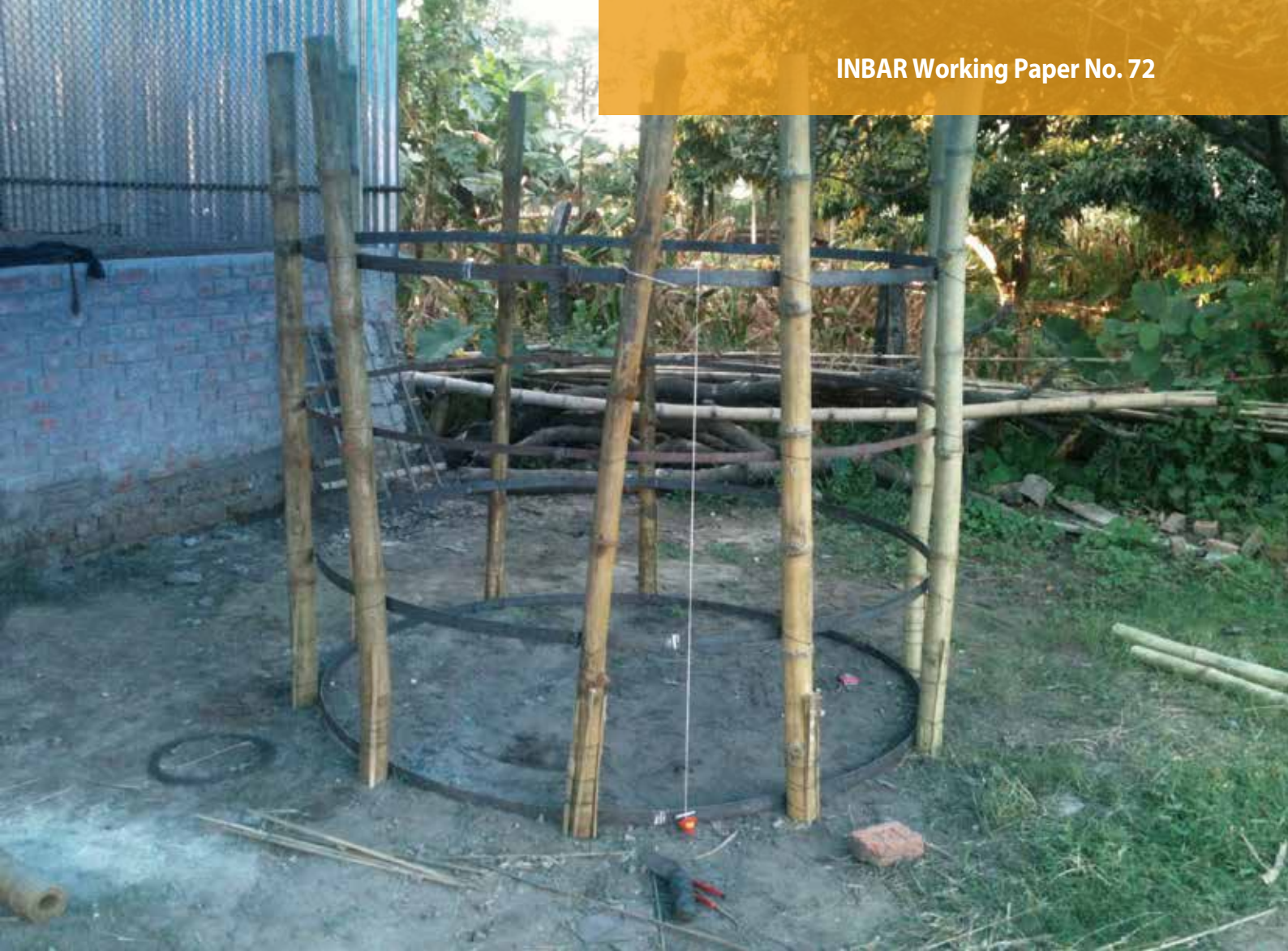
Figure 13: Positioning steel strips
