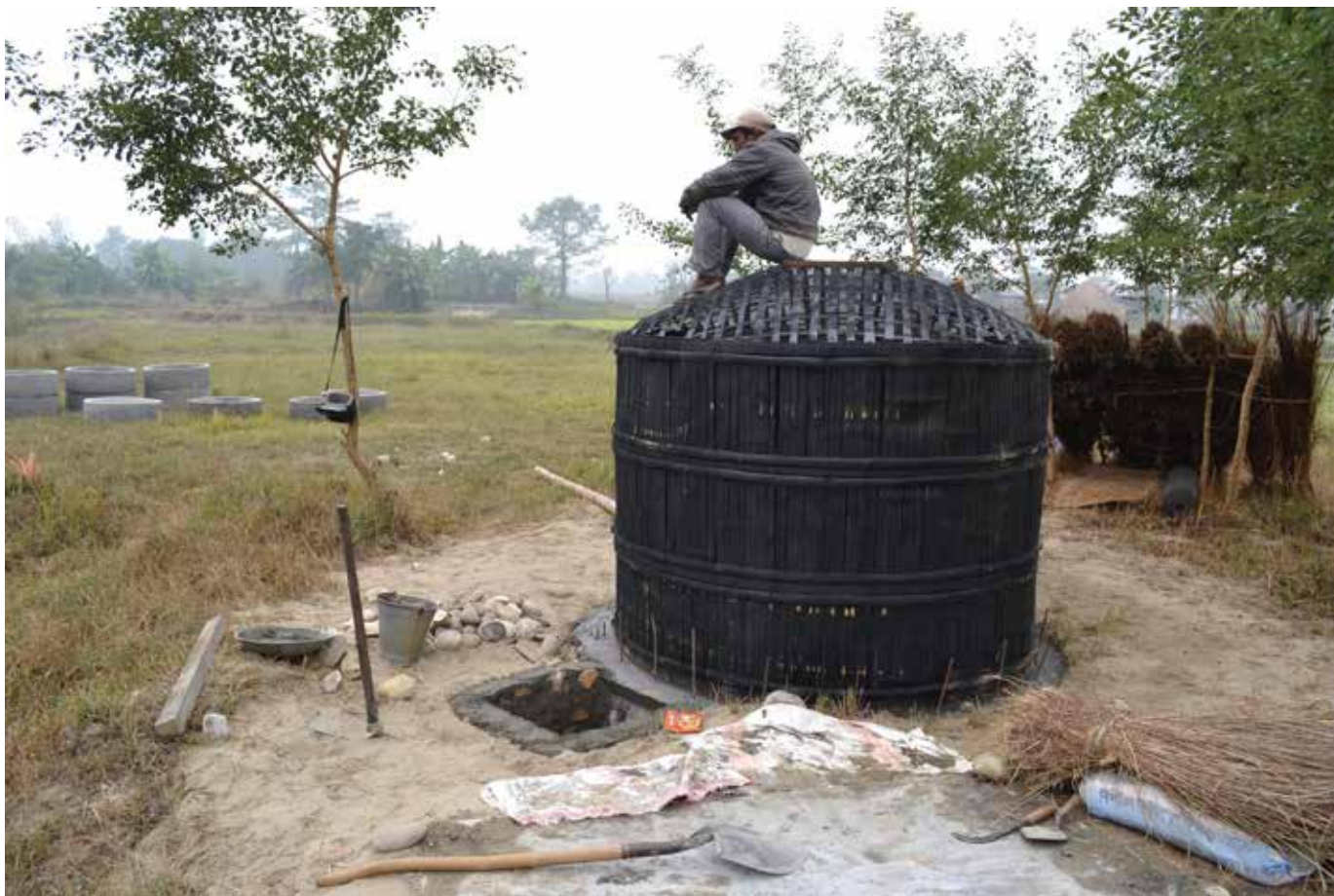
Figure 34: Tank ready for plastering
