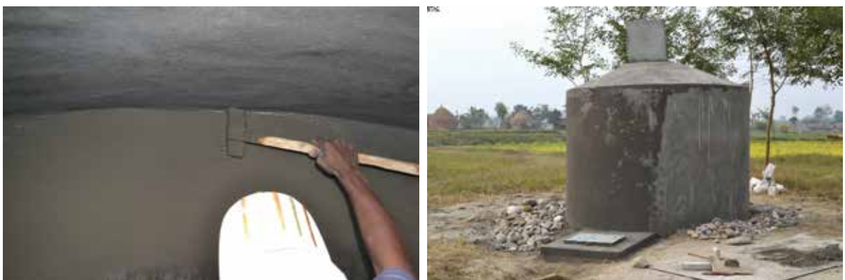
Figure 48: Cement water mixture interior application
