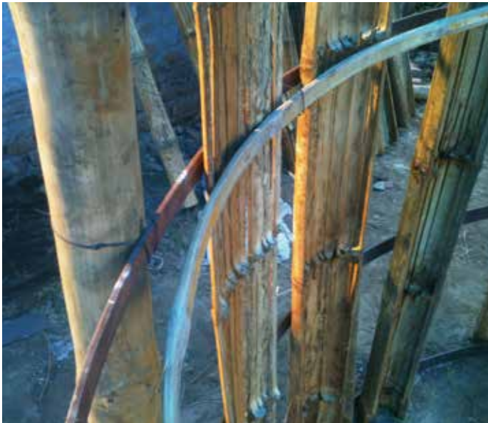
Figure 14: Fitting bamboo boards
