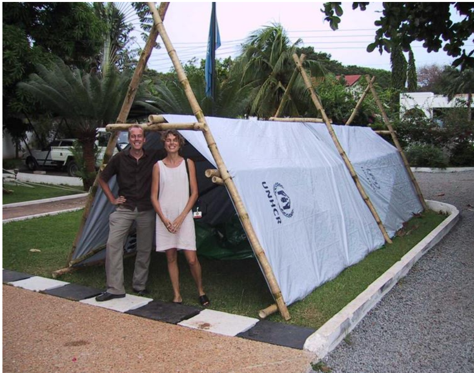
Picture 6: Second roof cover in place
