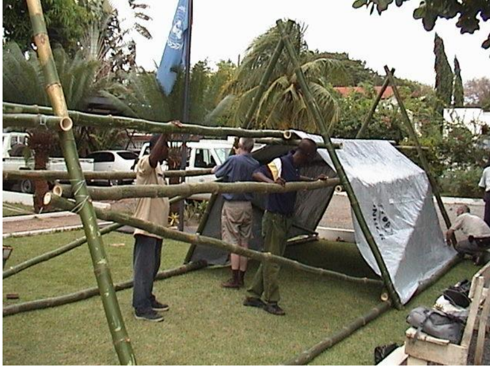
Picture 5: First roof cover in place
