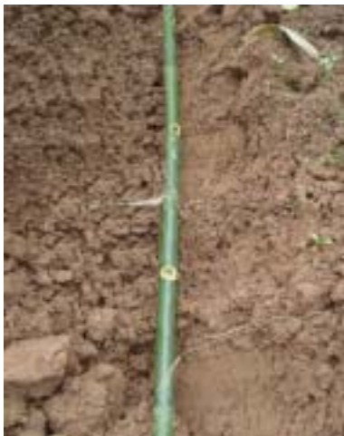
7. Dig a trench 5 to 10 centimeters deep with a horizontal bottom.
