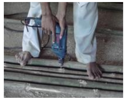
Drilling holes for treatment
