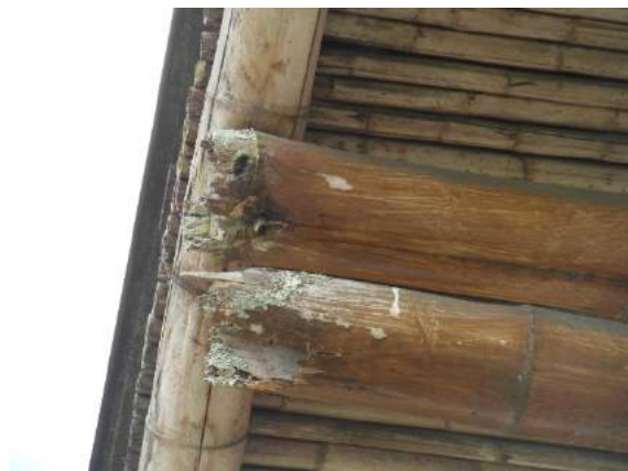
Figure 39: Rot to the exposed end of the bamboo in a roof, Costa Rica (Kaminski, 2016)
