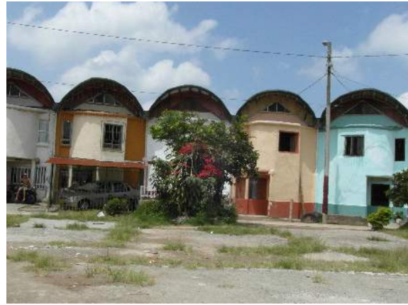
Figure 19: Post-earthquake engineered bahareque housing in Montenegro, near Armenia (Kaminski, 2016)
