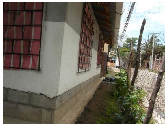
Figure 27: Cane and timber housing, El Salvador – complete. Note the upstand, damp-proof membrane and large overhang, all protecting the wall from moisture and rain (Kaminski, 2016)
