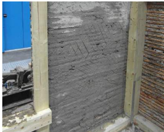
Figure 74: Maintaining a good bond between subsequent cement mortar render layers by roughening the previous layer while still setting (Kaminski, 2016)
