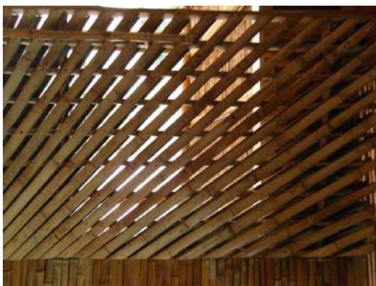
Figure 8: Reglilla (Colombia) or latillas (Ecuador): Laths of bamboo formed by cutting a large diameter culm along its length into strips (Kaminski, 2016)
