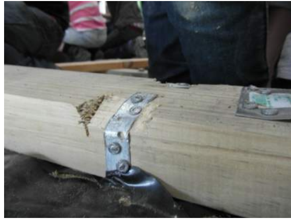
Figure 65: Photo of sole plate fixed to upstand with cast-in off-the-shelf steel straps, after nailing
