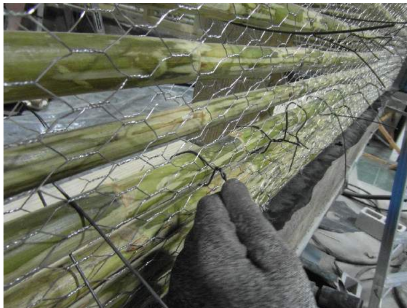
Figure 72: Installing steel wire through-ties to connect chicken mesh on both sides of the matrix
