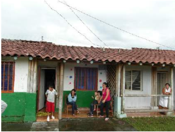
Figure 18: Post-earthquake engineered bahareque housing in Barcelona, near Armenia (Kaminski, 2016)
