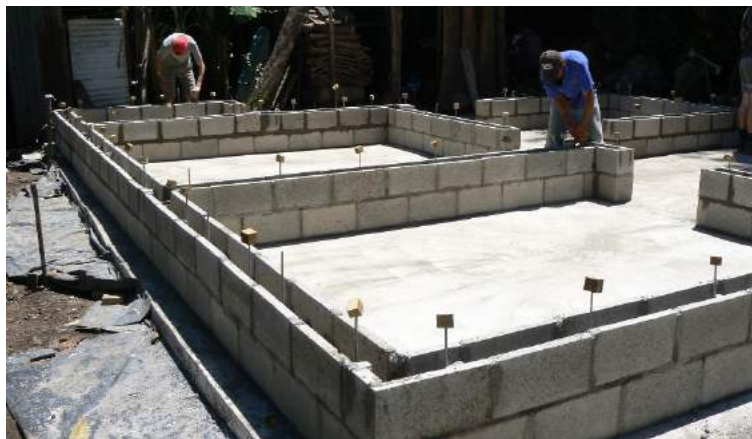
Figure 60: Example of simple upstand of engineered bahareque housing in El Salvador, consisting of two courses of reinforced blockwork, totalling 400mm high from the foundation
