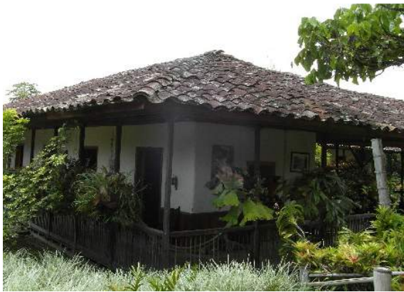
Figure 1: A well-constructed traditional rural bahareque house in Armenia, Colombia (Kaminski, 2016)
