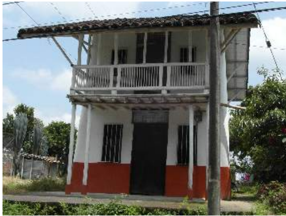
Figure 20: Post-earthquake engineered bahareque housing in Montenegro, near Armenia (Kaminski, 2016)
