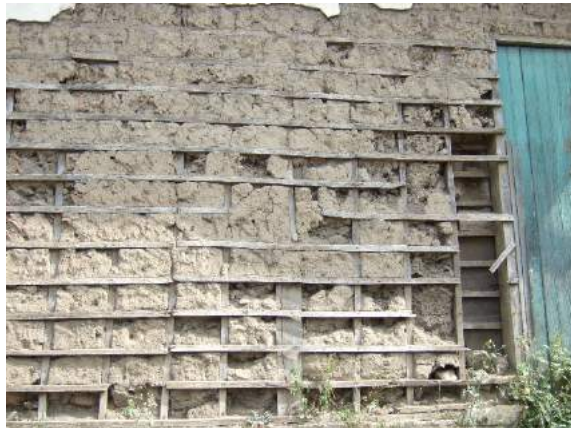
Figure 10: Timber hardwood battens nailed together to form a rectangular matrix spanning between larger vertical studs (Kaminski, 2016)
