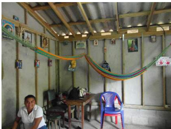
Figure 26: Cane and timber housing, El Salvador – complete (Kaminski, 2016)
