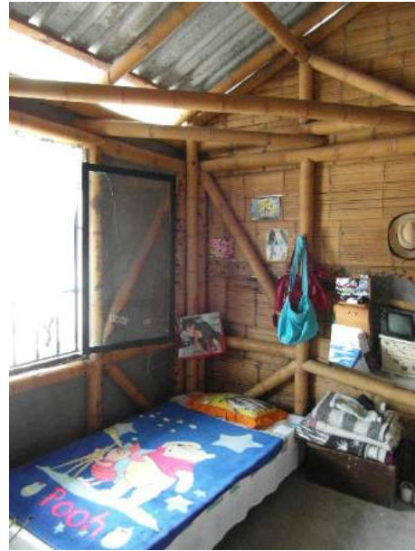
Figure 23: Post-earthquake engineered bahareque housing in Montenegro, near Armenia (Kaminski, 2016)
