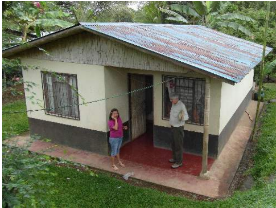
Figure 16: PNB house in Milano, Costa Rica – photo taken at 20+ years since construction (Kaminski, 2016)
