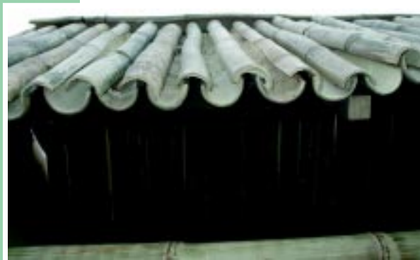
Bamboo roofing in Ghana
