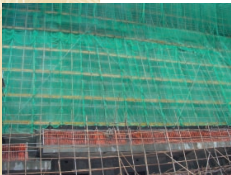
hybrid bamboo-steel scaffolding
