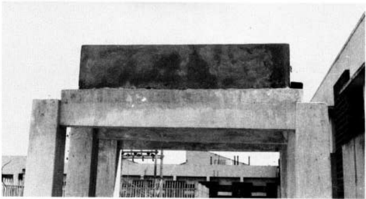
Fig. 6. Floor assembly with precast units (used for load test and durability).
