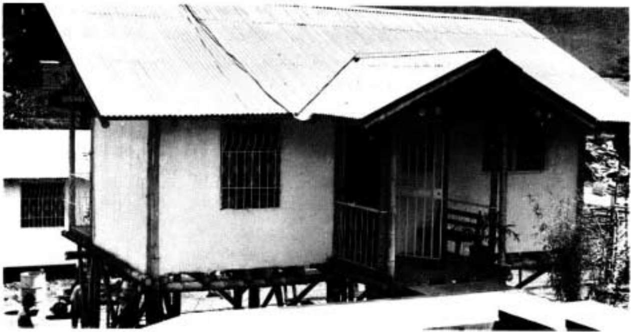
Fig. 2. Bamboo prototypes for rural construction in Costa Rica.
