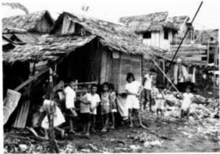
Fig. 6. External bamboo bracing (arrow).
