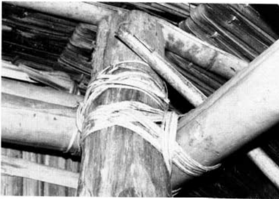
Fig. 2. Photograph of an undamaged bamboo tied connection.
