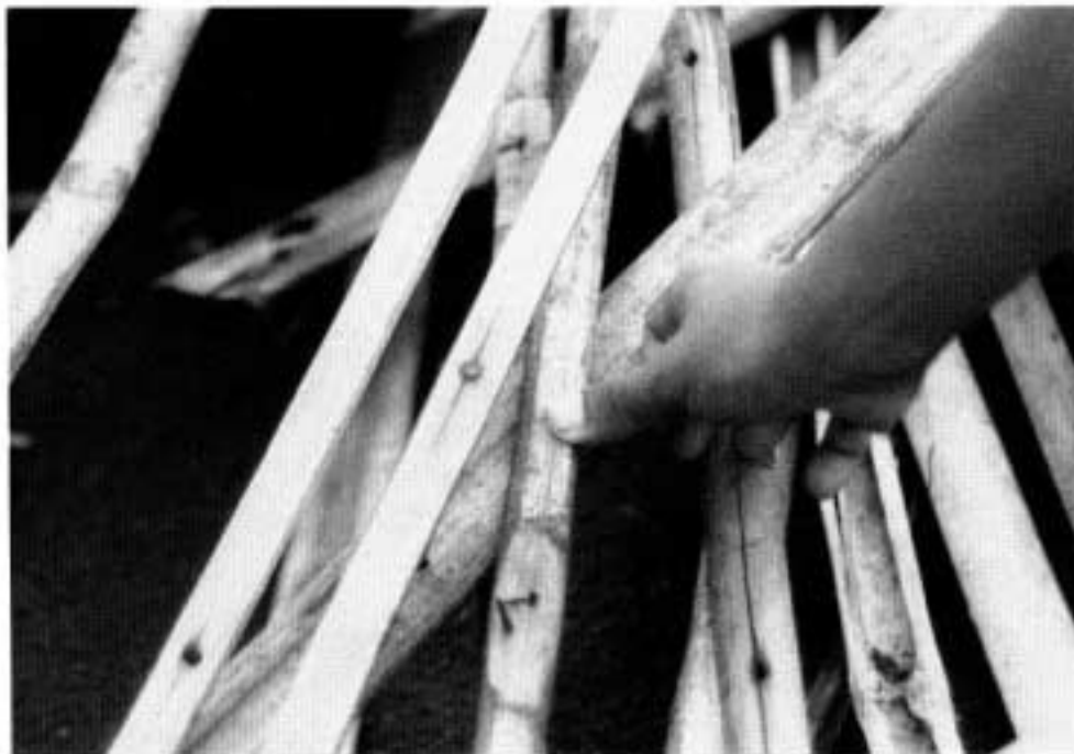
Fig. 3. Nailing of split bamboo pieces.
