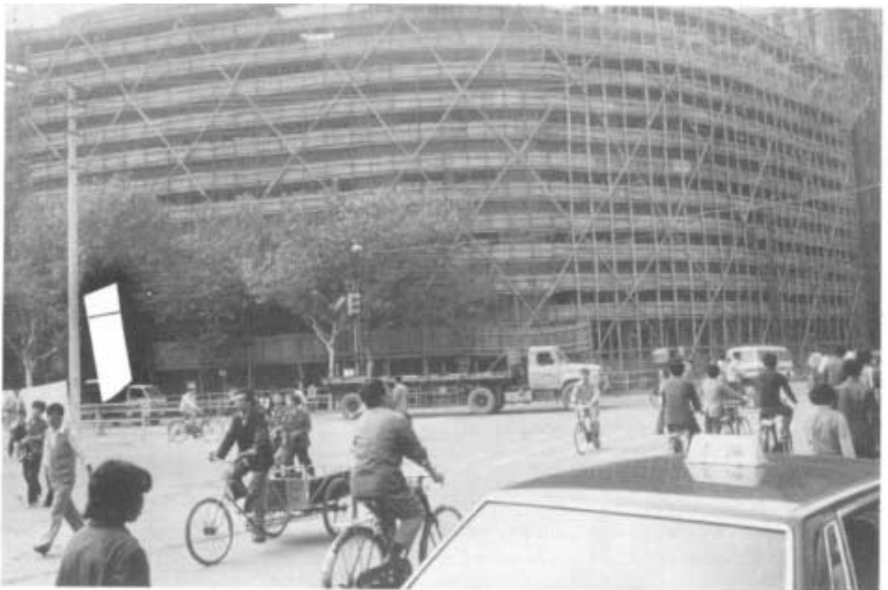
Fig. 5. Bamboo-scaffolding (Shanghai, 1985).
