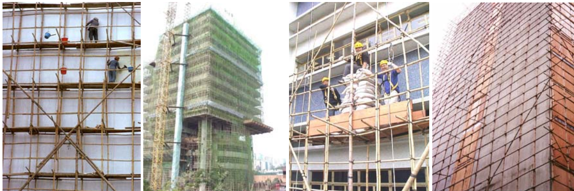
Bamboo scaffolding, Hong Kong
