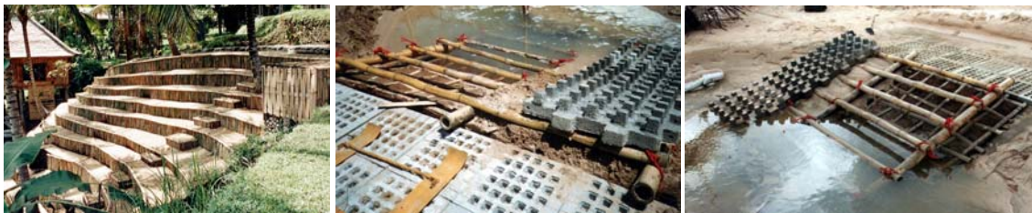
Bamboo retaining wall and bamboo-based erosion control system
