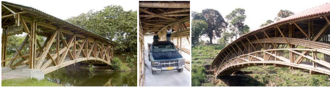
20m footbridge and 52m bamboo road bridge, Colombia
