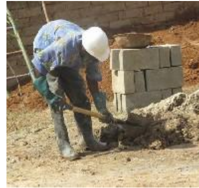
Plate 32: A worker working with protective gear
