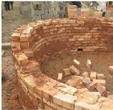
Plate 6: Smoke exit opening
