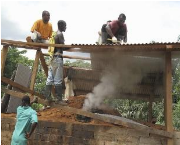
Plate 17: Roofing of shelter
