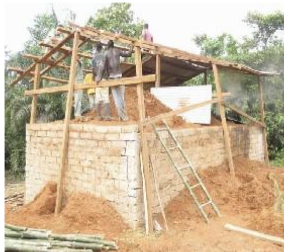
Plate 18: Kiln shelter construction
