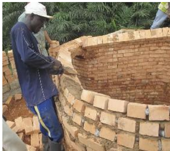
Plate 4: Brick laying with gravels providing support at the clay mortar joints
