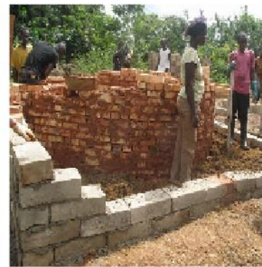
Plate 7: Side view showing the brick kiln and the cement wall
