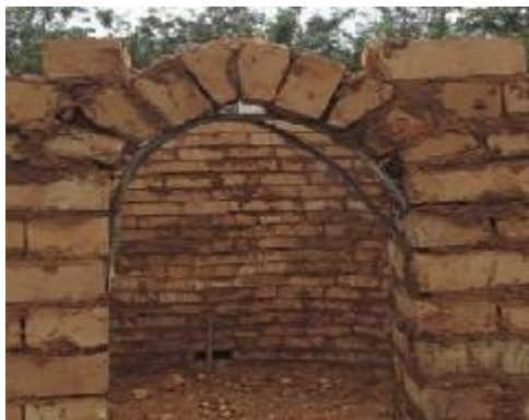
Plate 13: Sticks used for supporting the arc of the doorway
