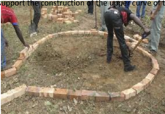
Plate 11: Arrangement of the first layer of bricks
