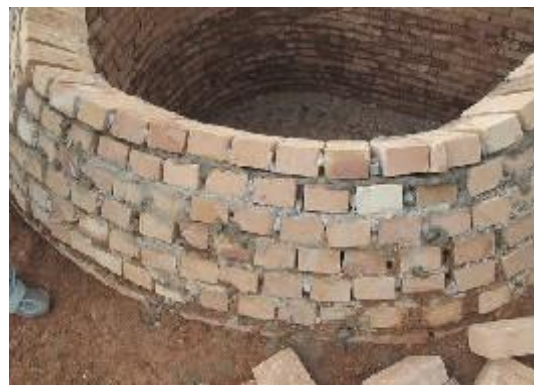
Plate 14: Gravels used for supporting the mortar joints
