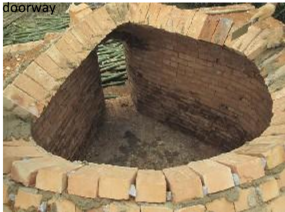
Plate 2: Aerial view of an uncompleted kiln
