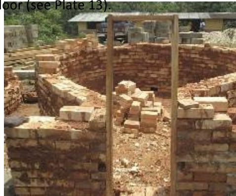
Plate 12: Door frame for shaping the doorway
