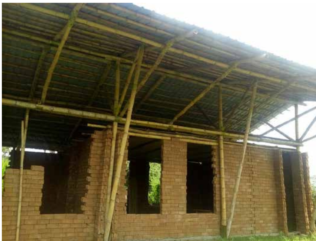
Fig. 20: Use of bamboo as roof trusses at Moi Siongiroi Girls School in Bomet County
