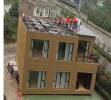
光伏安装 PV Panel Installation
