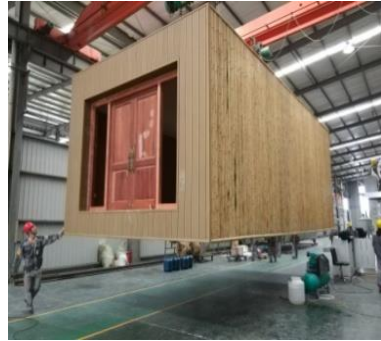
房屋起吊 House Lifting UP
