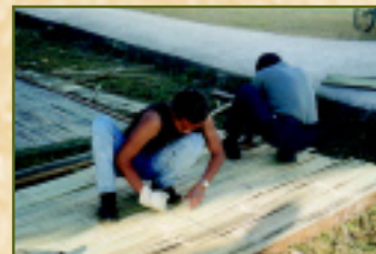
Constructing wall panels of bamboo on wooden frameworks in Nepal
