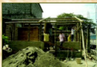
Constructing the framework of the hybrid house
