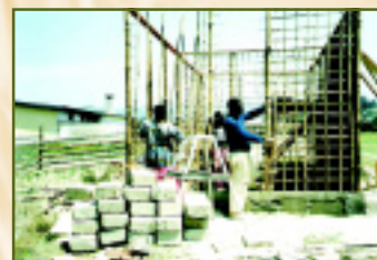
Preparing the framework for plastering, Tanzania
