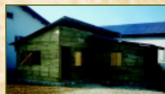
The finished house before plastering
