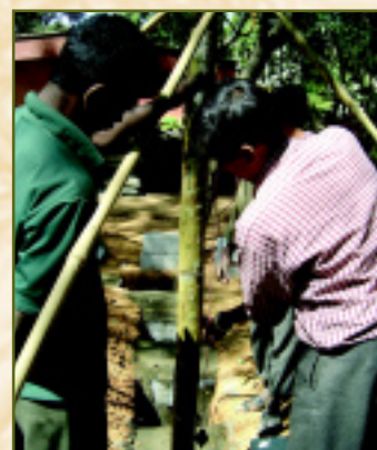
Installing the uprights, Bangalore, India
