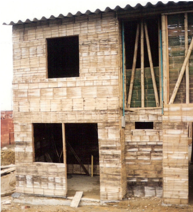
Left: Split bamboo mats nailed onto bamboo frames at 'Bambusa' in Colombia: the first housing project to be designed in accordance with Chapter E.7. Architect: Jaime Mogollón; Engineer: Samuel D. Prieto. Right: Engineered bahareque house on a shake table at Universidad de Los Andes. Its seismic performance was excellent. Credit: David Trujillo.
