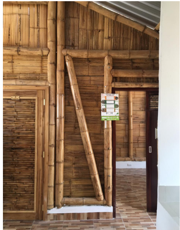
A detail from inside the house. Credit: INBAR.
