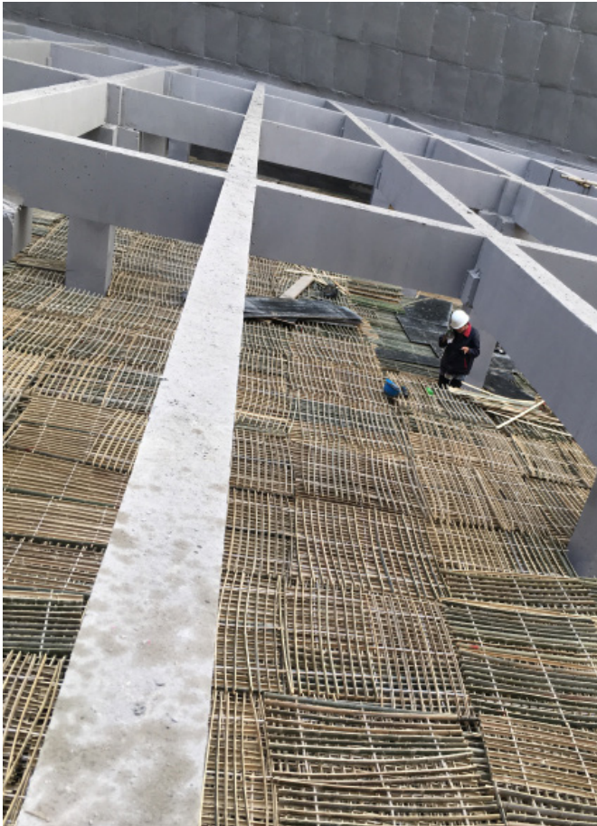
Bamboo grid packing being installed at the Dongfeng Power Plant, one of 80 companies in China to use this equipment. Credit: Ma Xinxin et al.
