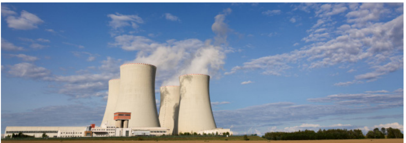
In recent decades, cooling towers of power plants have been lined almost exclusively with PVC grid packing.
