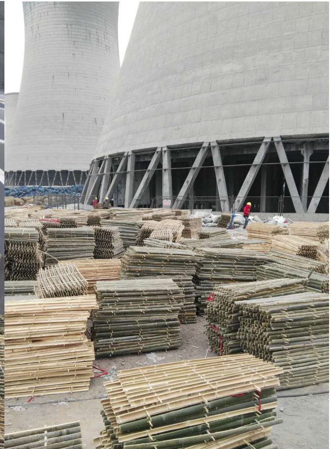
Bamboo grid packing being installed at the Dongfeng Power Plant, one of 80 companies in China to use this equipment. Credit: Ma Xinxin et al.
