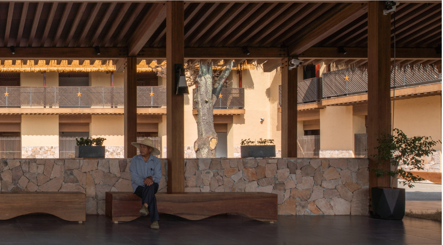
The bamboo glulam structure in No. 4 Yard, Lixiang Village is a space shared by villagers and tourists. Credit: Timeraw Studio.
