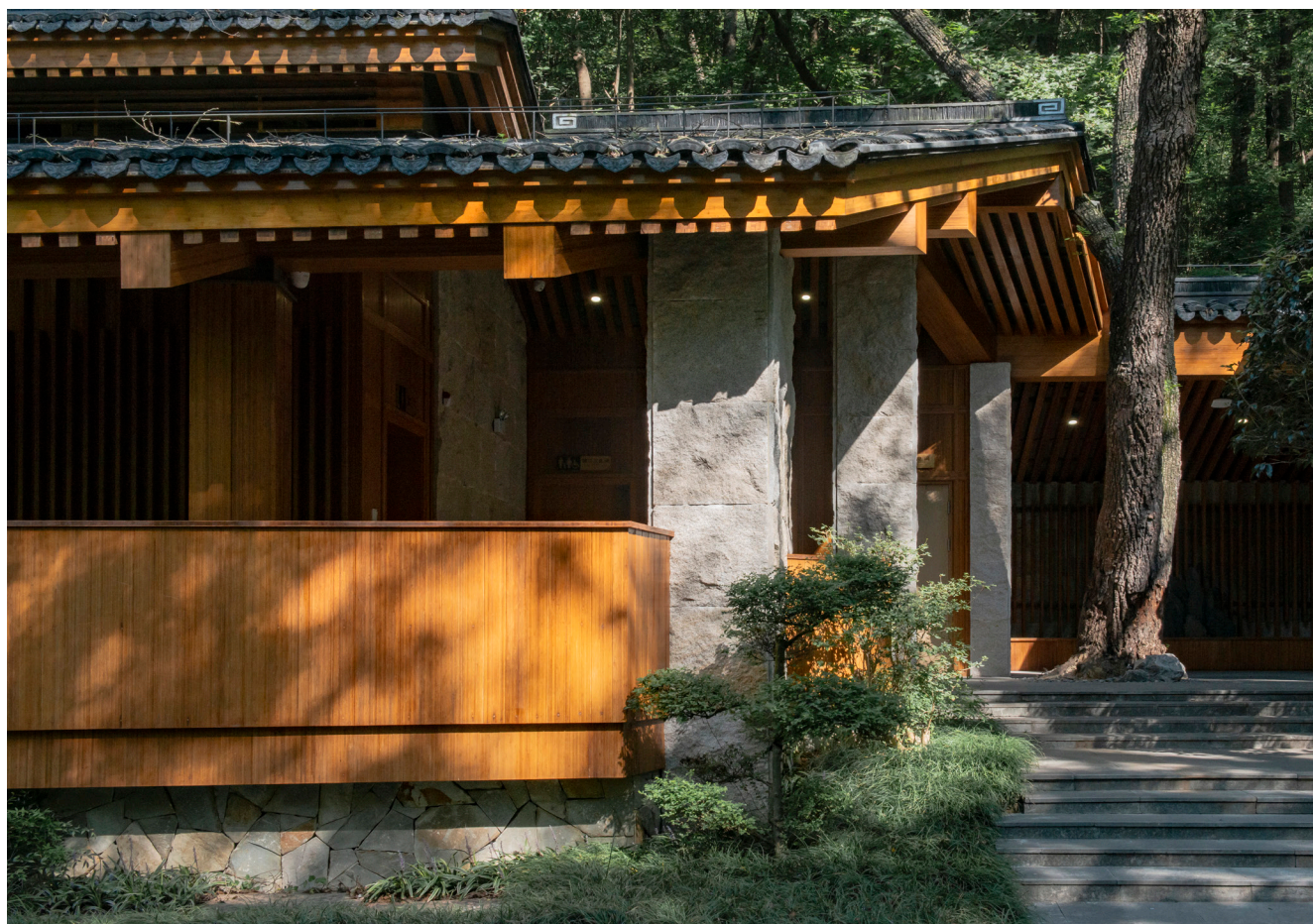
Nanjing Qixia Mountain Scenic Area Tourist Station. As an earlier project by ATA Studios, the bamboo here is mainly decorative, not structural. Credit: Timeraw Studio.
