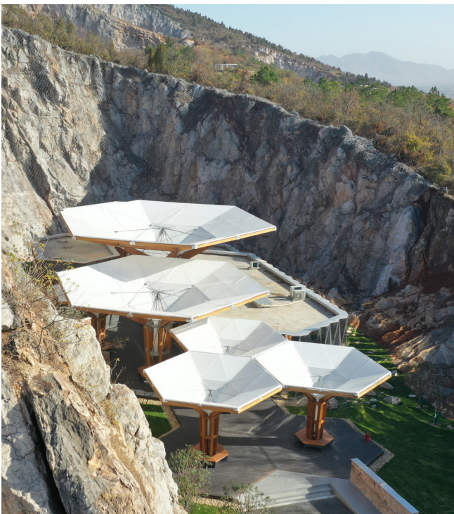
Details from the bamboo glulam structure Tangshan Pit Camp Tourist Center, which is situated in an old mining site. The largest bamboo 'mushroom' roof has a diameter of 19 metres. Credit: Timeraw Studio.
