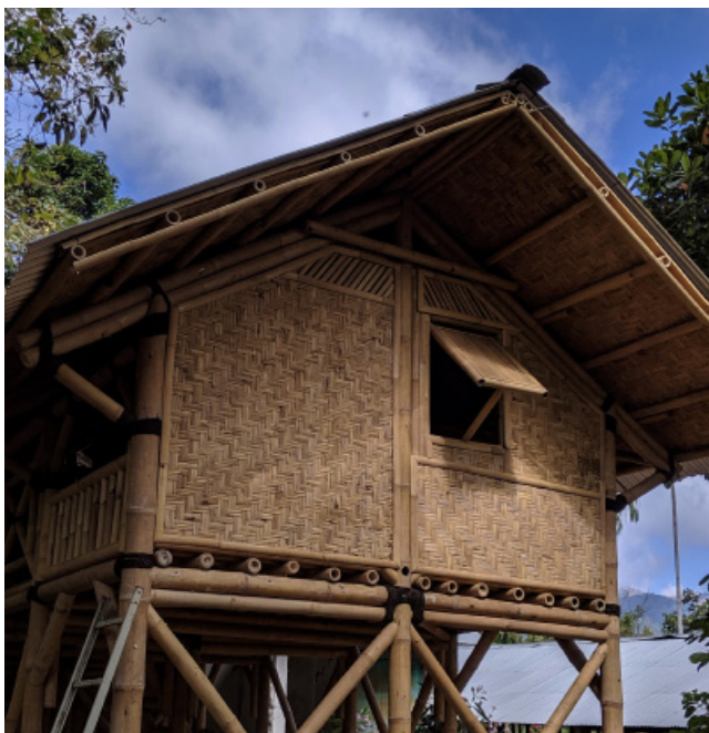
In BRU Volume 2 Issue 1, structural engineering firm Ramboll described their work building earthquake-resilient houses with round bamboo. Credit: Ramboll UK.
