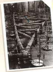
↑ TEST ON TRUSS, three span 8 meters
