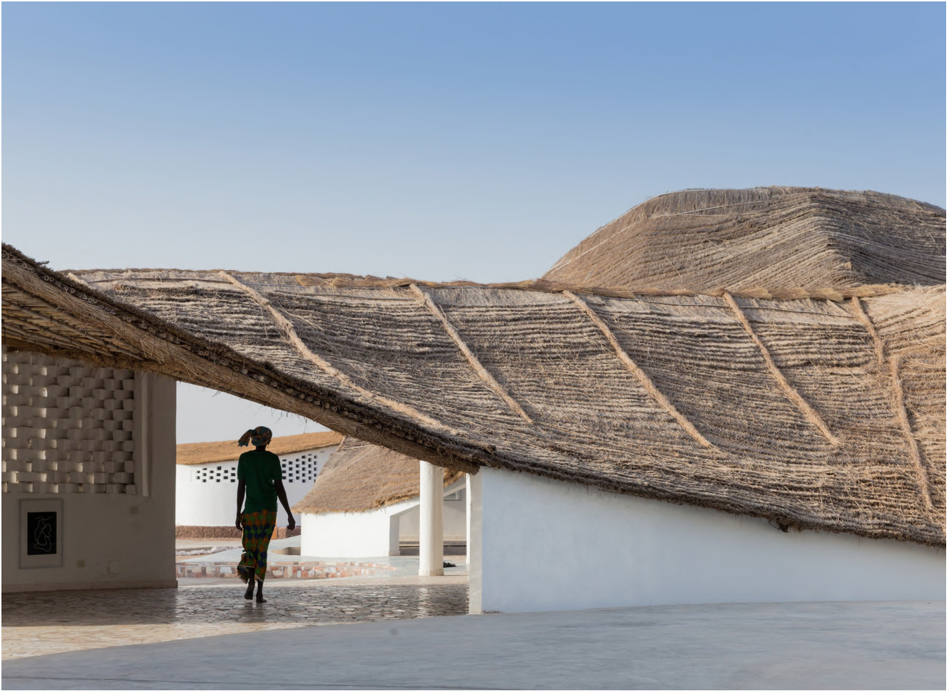
The award-winning cultural centre 'Thread' in Sinthian village, Senegal, designed by Japanese architect Toshiko Mori, was constructed using local materials including bamboo. The centre provides a unique environment for activities, including an agricultural programme run by non-profit organisation Le Korsa. Credit: Iwan Baan / Le Korsa.
