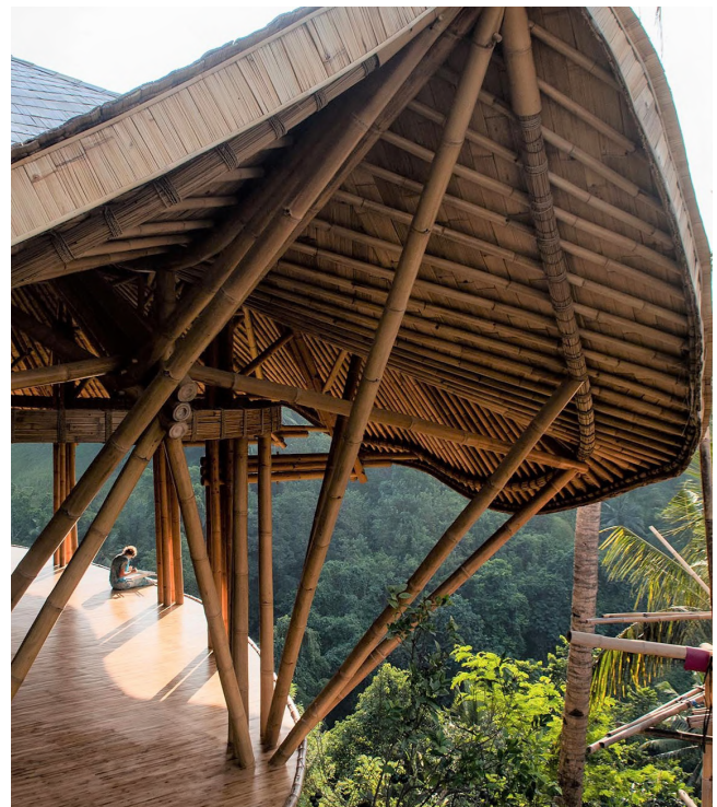
The new open-plan tea house in Bali is designed entirely from bamboo. Credit: Valentina Gebrie.
