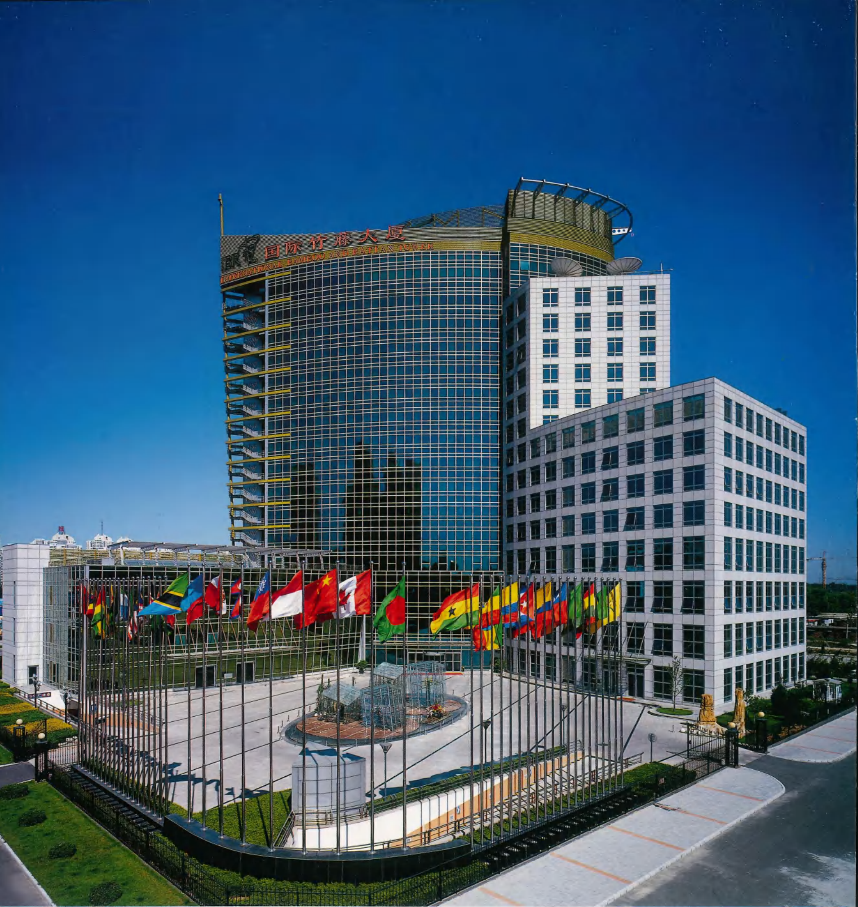
The International Bamboo and Rattan Tower (photo: September 2004)
