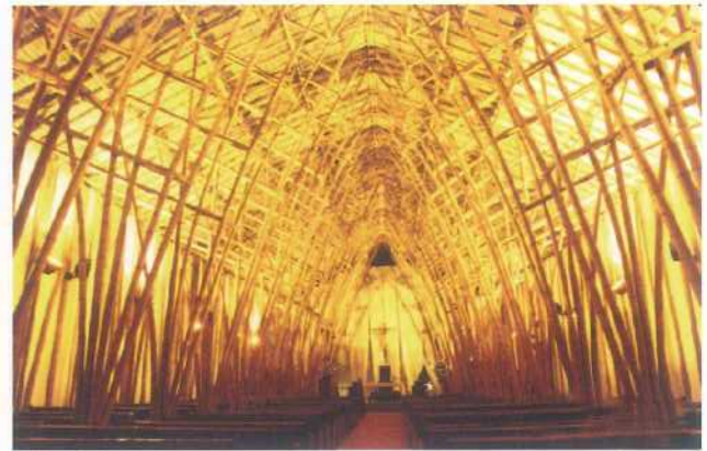
INBAR extends advanced bamboo construction technologies in Colombia to other South American Countries. Top left: Top grade bamboo residence of South America; top right: a bamboo structure in Church Simon Velez of Colombia.
