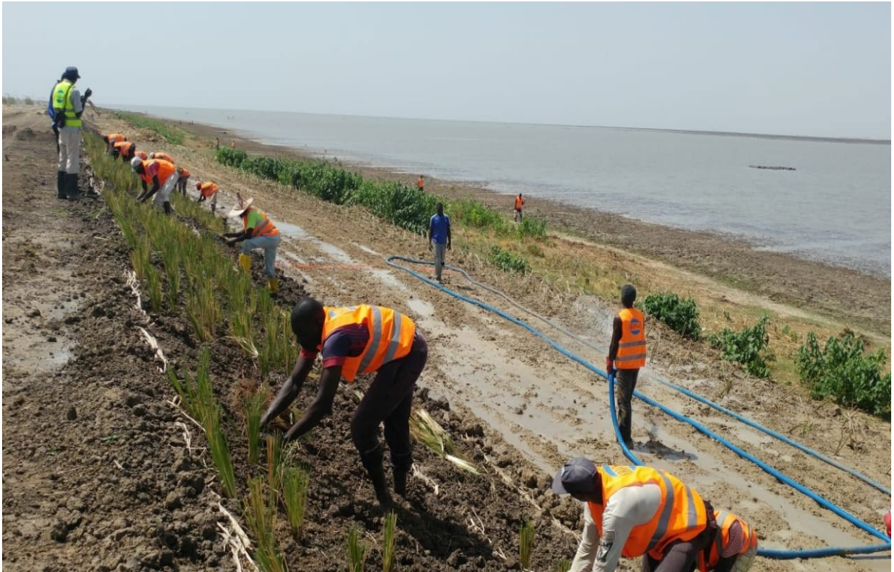
2017, The banks of Lake Maga in the Far-North Region are being restored thanks to revegetation of Vétiver and Ipomea. @ABIOGeT
