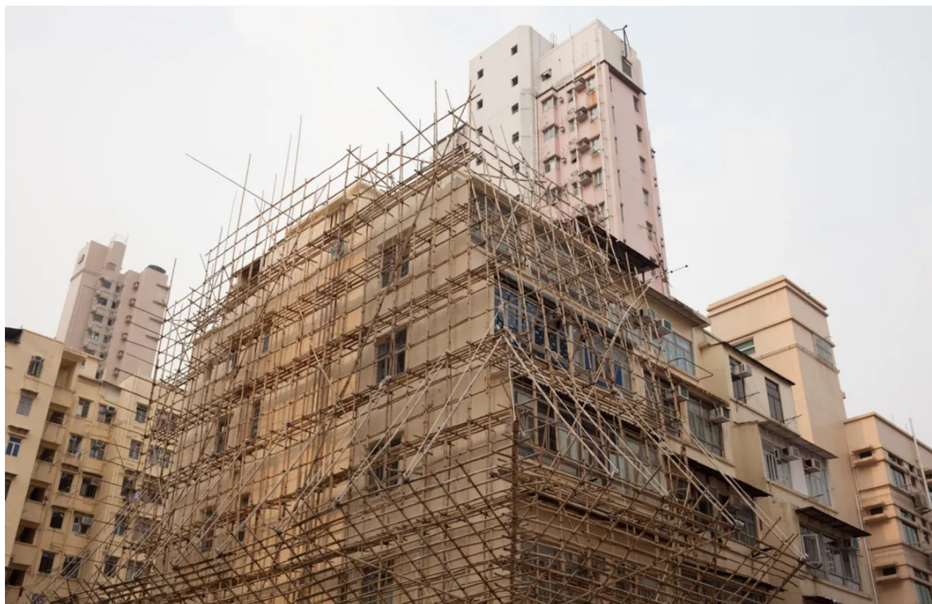
Bamboo scaffolding erected around a building in Hong Kong. Credit: iStock.
