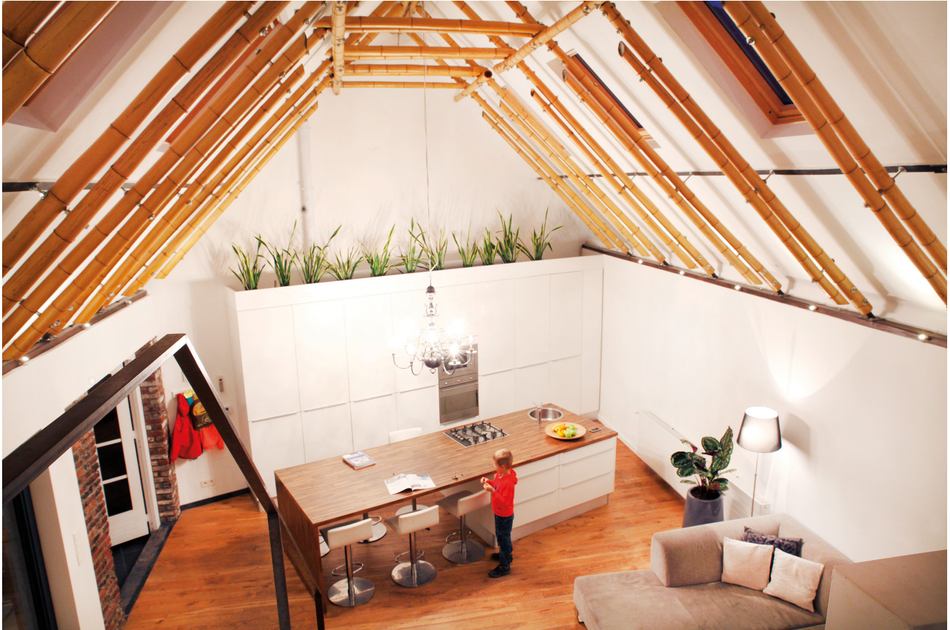
One of the few examples of the structural use of bamboo stem in a permanent structure in Europe. This private home was designed by architect Sven Mouton in Ghent, Belgium. Credit: Sven Mouton
