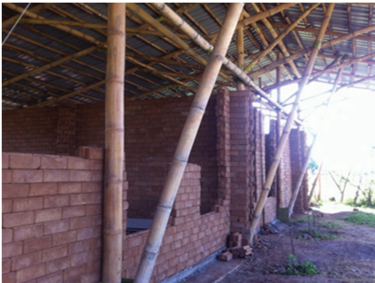
Roof trusses made from bamboo culms - at Moi Siongiroi Girls Secondary School
