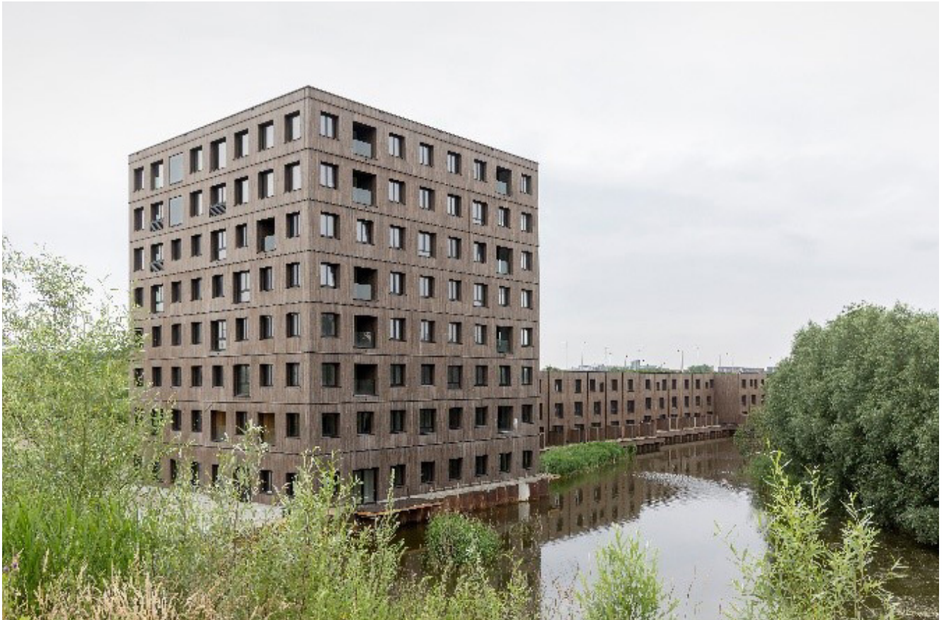
The multi-story residential building Switi in Amsterdam, designed by HoH Architects, is a compelling example of a building that consistently applies bio-based alternatives. Credit: Marcel van den Burg.
