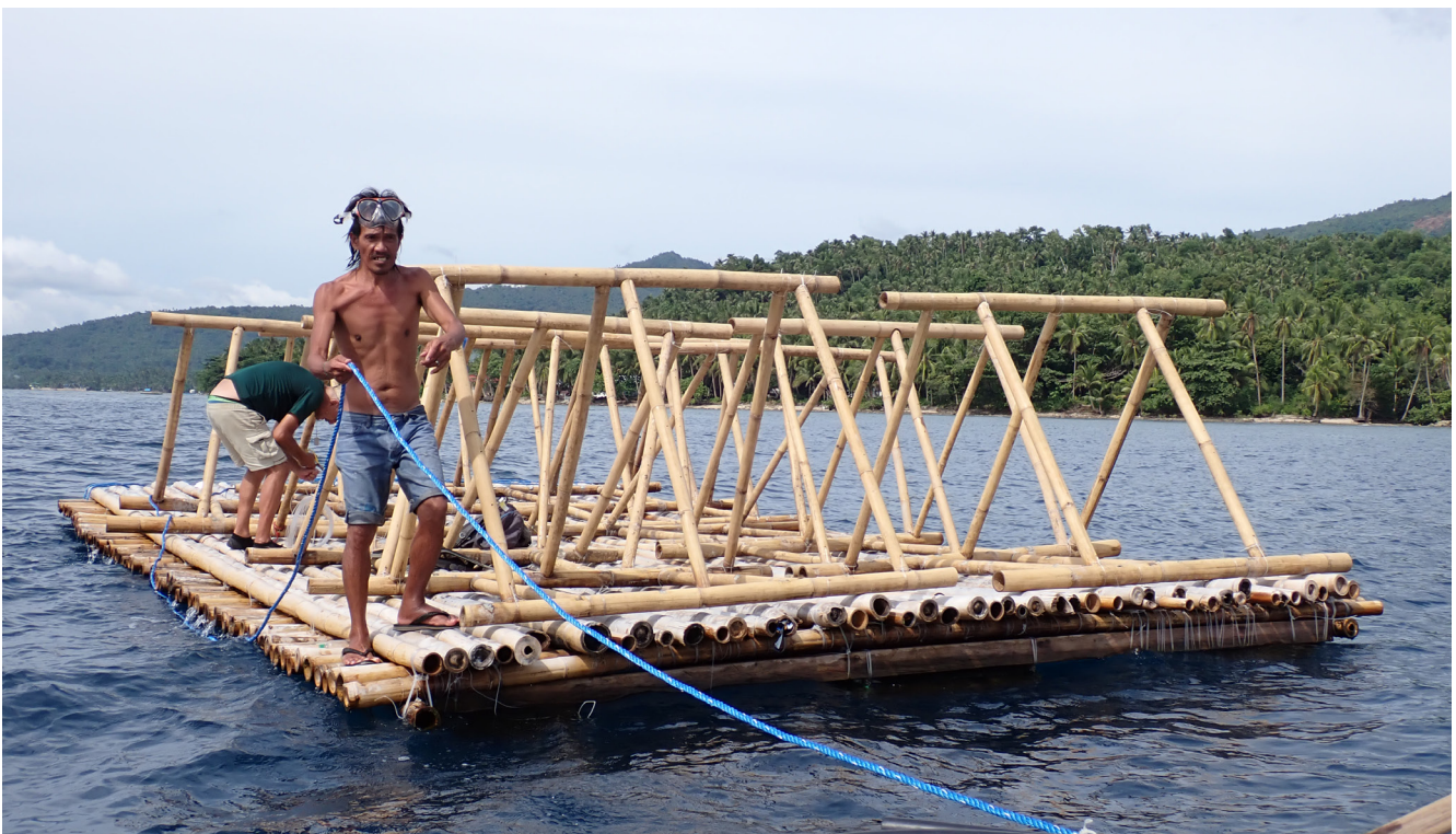
Preparing the bamboo structures for lowering to the seabed. Credit: Anthony Into.
