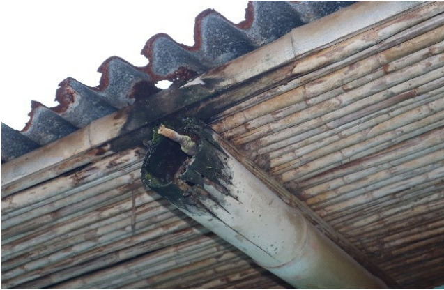
Left: Bamboo rafter rotten where exposed to rain in Costa Rica. Right: Bamboo column rotten where exposed to driving rain in Colombia. Credit: Sebastian Kaminski.
